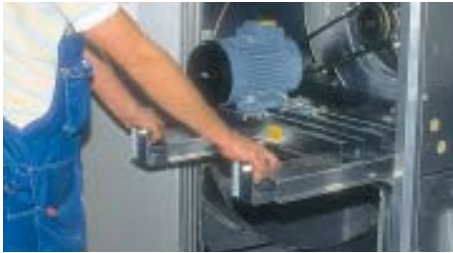
Withdrawable components and large inspection doors make maintenance easy.
