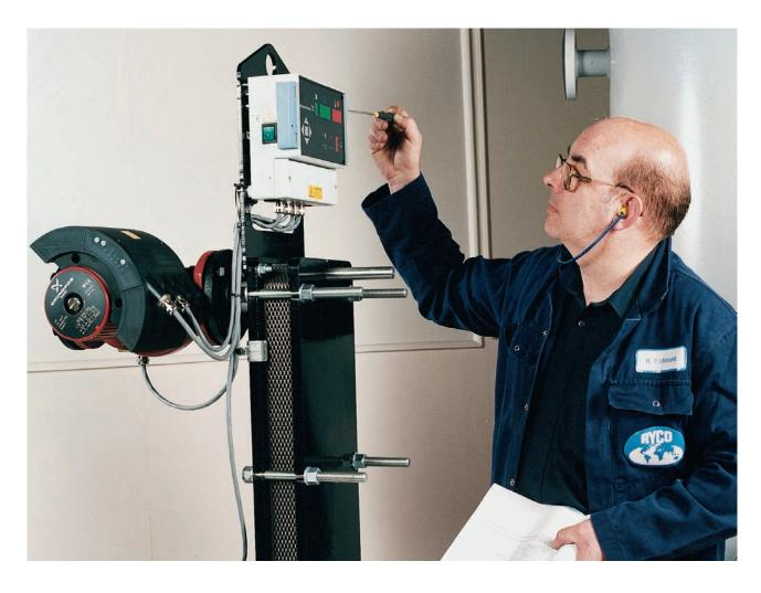
The Vari-E-Breeze controller measures the temperature in the secondary pipework (using a sensor in the flow)
